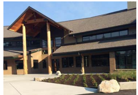
John D. “Bud” Hawk Elementary at Jackson Park is located on the same site as the original school building, which was built in 1967.
