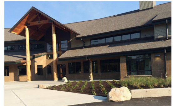
John D. “Bud” Hawk Elementary at Jackson Park is located on the same site as the original school building, which was built in 1967.
